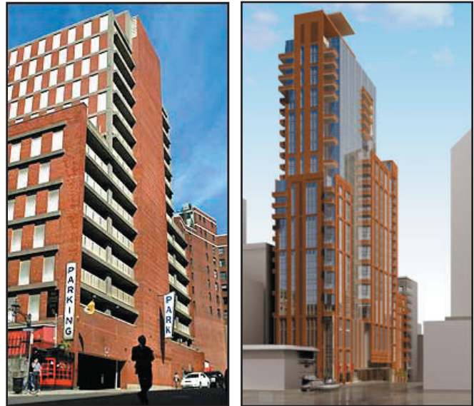
Developers will raze a parking garage (left, Globe photo) on Province Street to build a 31-story tower with condos, retail space, and a restaurant (right, Abbey Group).
